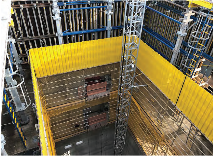
ABOVE: A view into the building core, showing the safe access from the construction hoist to the Doka automatic climbing formwork
