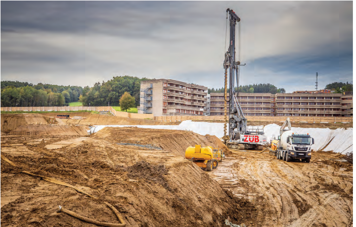
ABOVE AND BELOW: Züblin Spezialtiefbau was contracted to install 1,310 piles for the foundation of a new general hospital in Oberwart, Austria. To complete this task, the company used a Liebherr LB 28 drilling rig equipped with the LIPOS positioning system. The machine was supported on site by a Liebherr THS 110 concrete pump.
