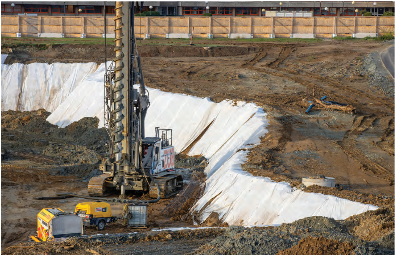
ABOVE AND BELOW: Züblin Spezialtiefbau was contracted to install 1,310 piles for the foundation of a new general hospital in Oberwart, Austria. To complete this task, the company used a Liebherr LB 28 drilling rig equipped with the LIPOS positioning system. The machine was supported on site by a Liebherr THS 110 concrete pump.
