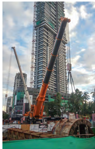
ABOVE: The AC 1000-9 has a 1,200-t capacity. In this project, the crane had to be equipped with its full 228-t counterweight for a boom length of 30 m.
